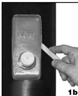
Trace outline of housing onto well casing.
