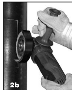
Or use a 4 1/2" hand grinder to cut opening.
