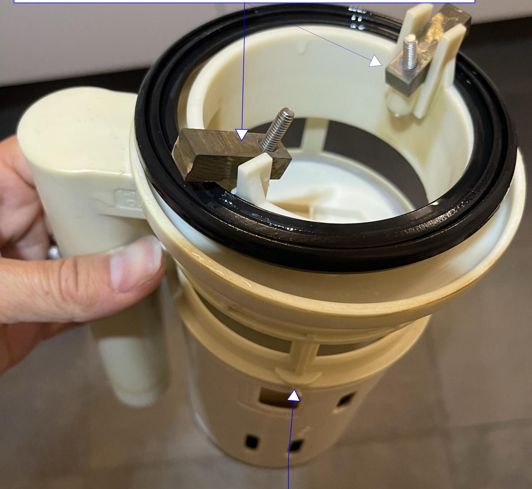
OPTION 1: TWIST OFF TO LEFT (CCW) AT UPPER SECTION TO REMOVE IF AT ALL POSSIBLE. IF NOT, GO TO OPTION 2
